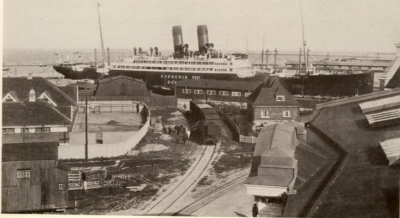
S/S Frederik VIII of 11850 tons in the dry dock for repairing
