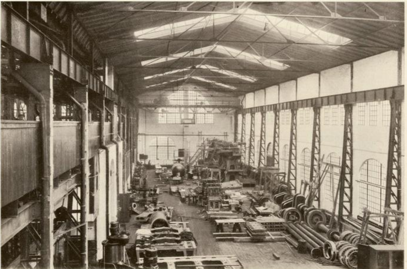
Machine shop: Diesel Engine erecting shop
