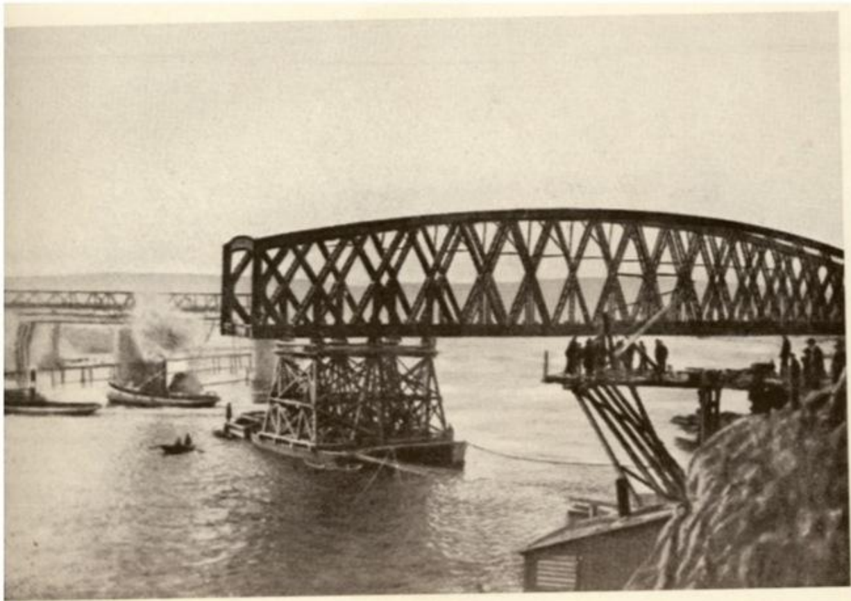
Railway bridge, Nordre Älv, Sweden
